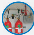
CO2 Fire Protection Smoke & Heat Sensors Fire Wire Drop-Valve
